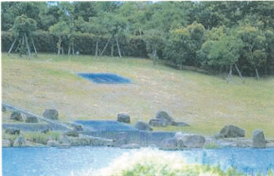
Outlet of Souzou-no-mori Detention Pond
