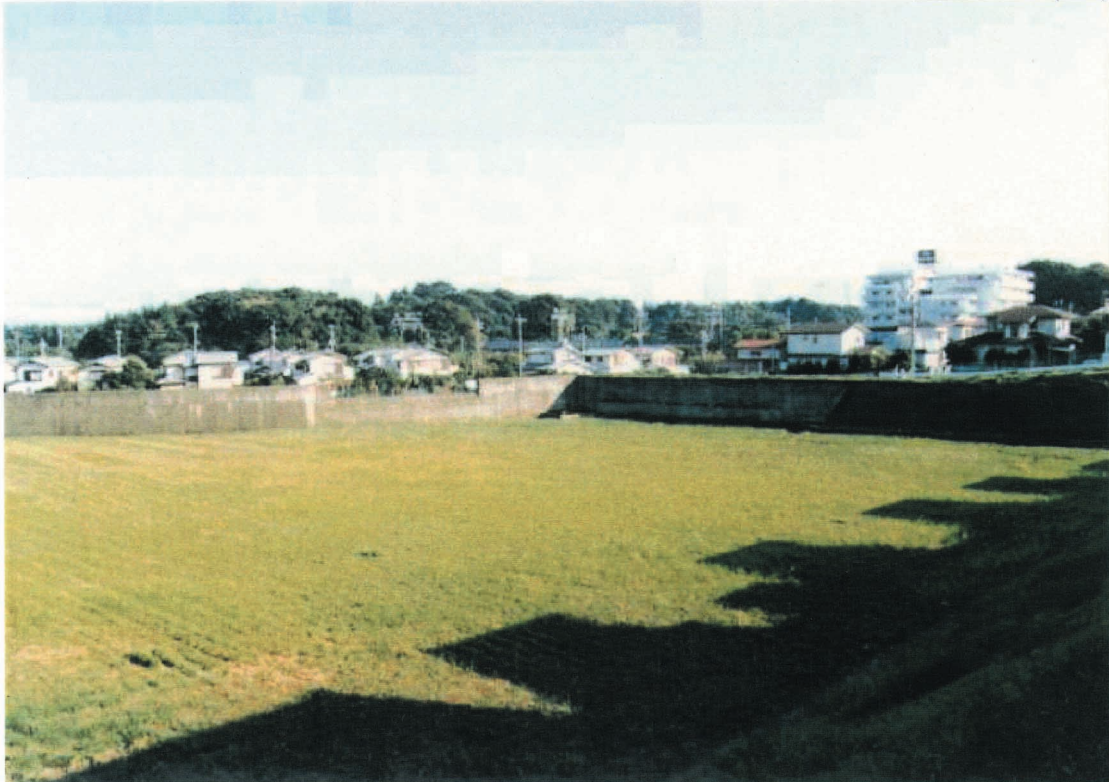
Hinatayama Detention Pond, Yokohama City, Kanagawa (Built in 1976)
