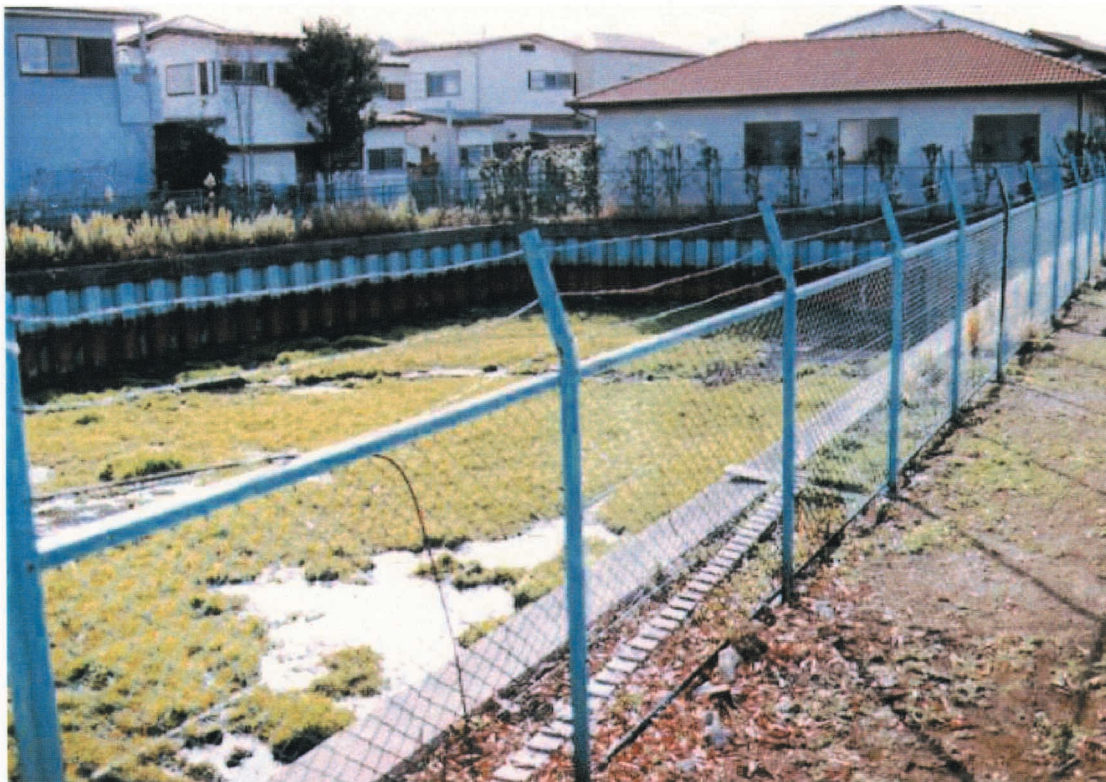
Fujigaoka Detention Pond, Kasukabe City, Saitama (Built in 1977)
