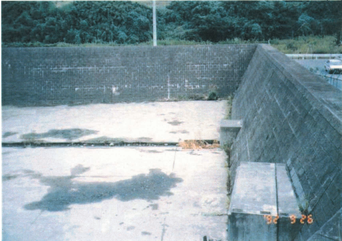
Miho Detention Pond, Yokohama City, Kanagawa (Built in 1970s)
