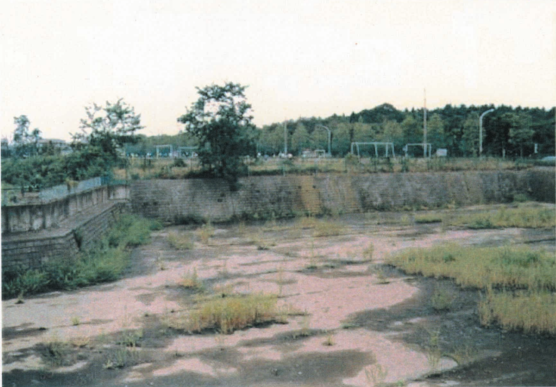
Turuma-1 Detention Pond, Machida City, Tokyo (Built in 1970s)
