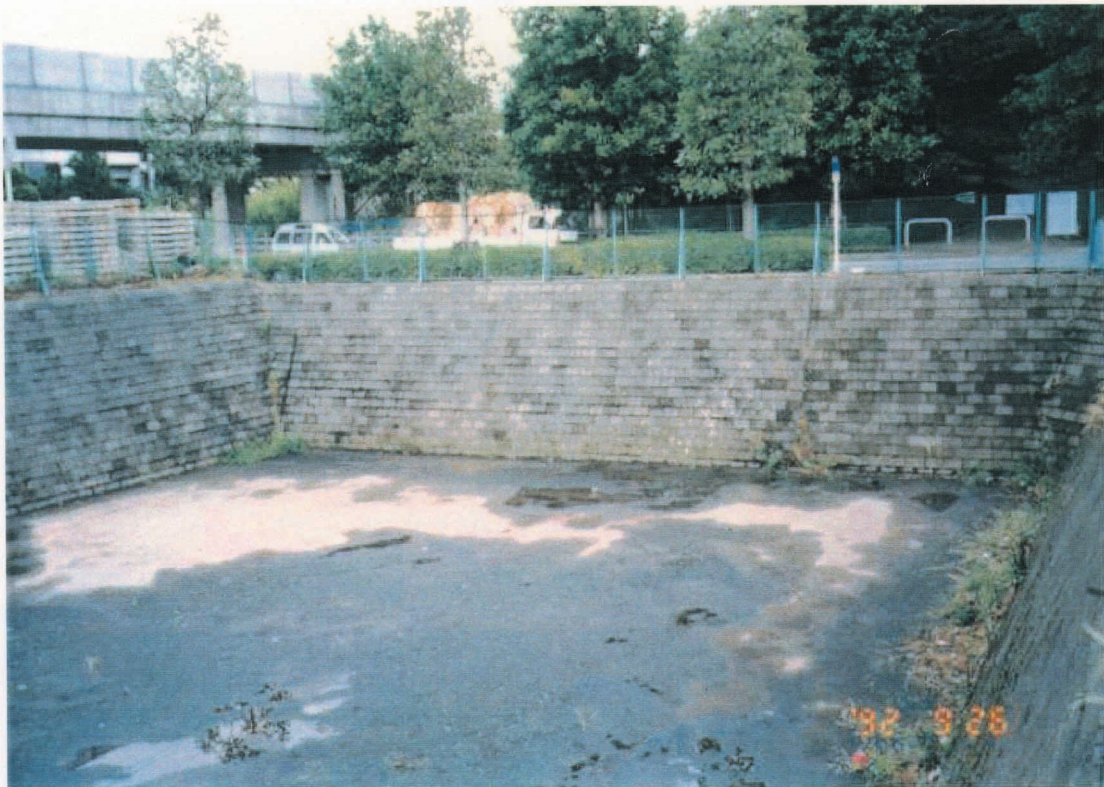
Turuma-2 Detention Pond
