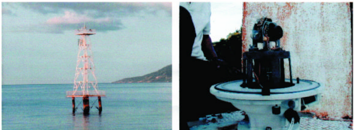
Photo 4.1.5 Leading light tower and lamp
