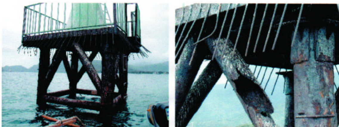
Photo 4.1.2 Typical photograph of the pile structure
