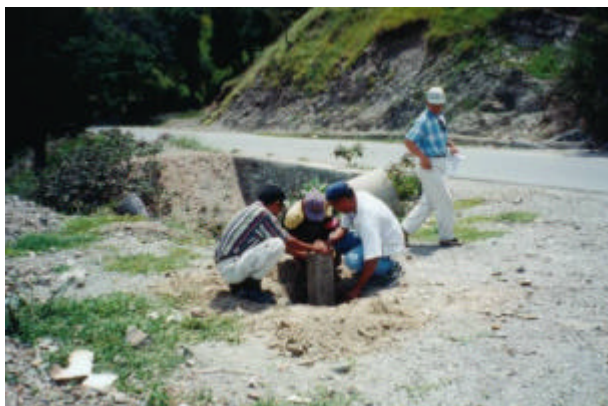
Establishment of concrete monument at JICA-2 point
