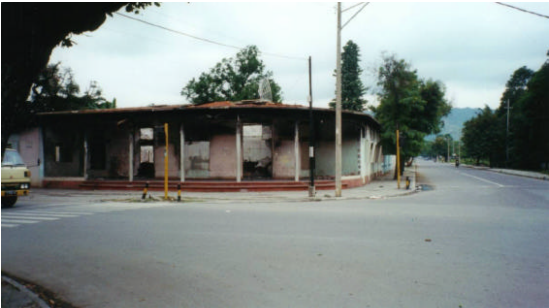
The house destroyed and burnt in September 1999 in Dili City
