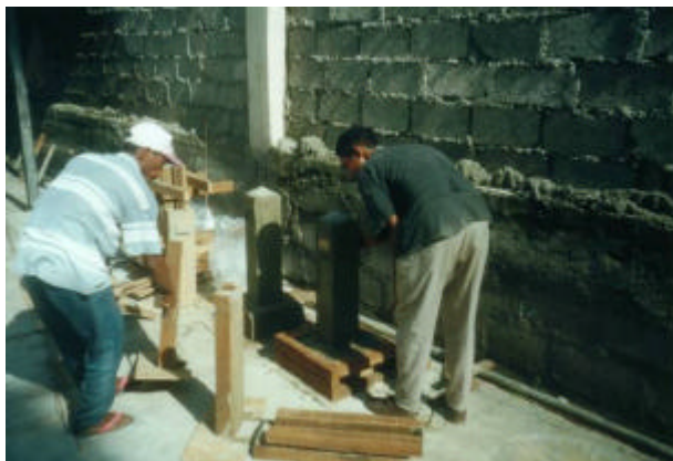
Preparation of concrete monuments for GPS points
