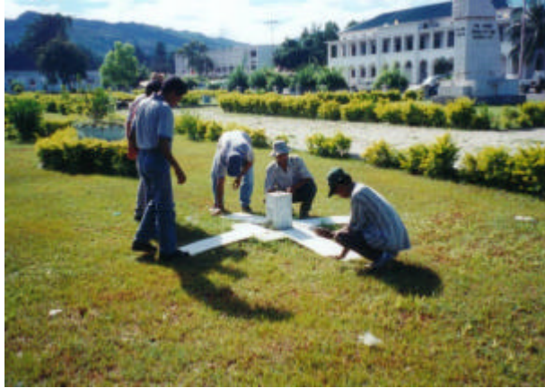
Establishment of pre-mark at TTG-0157 (In front of the main office of the UNTAET)
