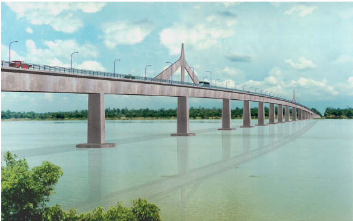
View of the Main Bridge from the Thailand side
