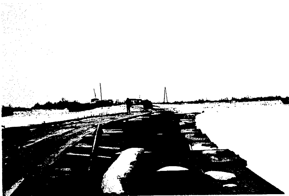
Pontoon bridge over Syrdarya River (Winter)
