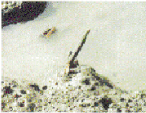
Photo 38 Damage by Crabs
