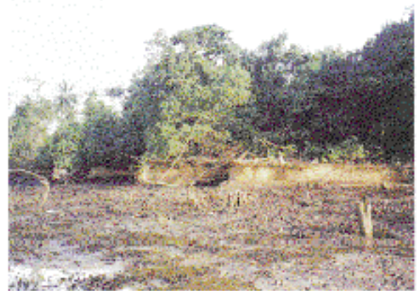
Photo 15 The eroded coastline at Bengkalis
