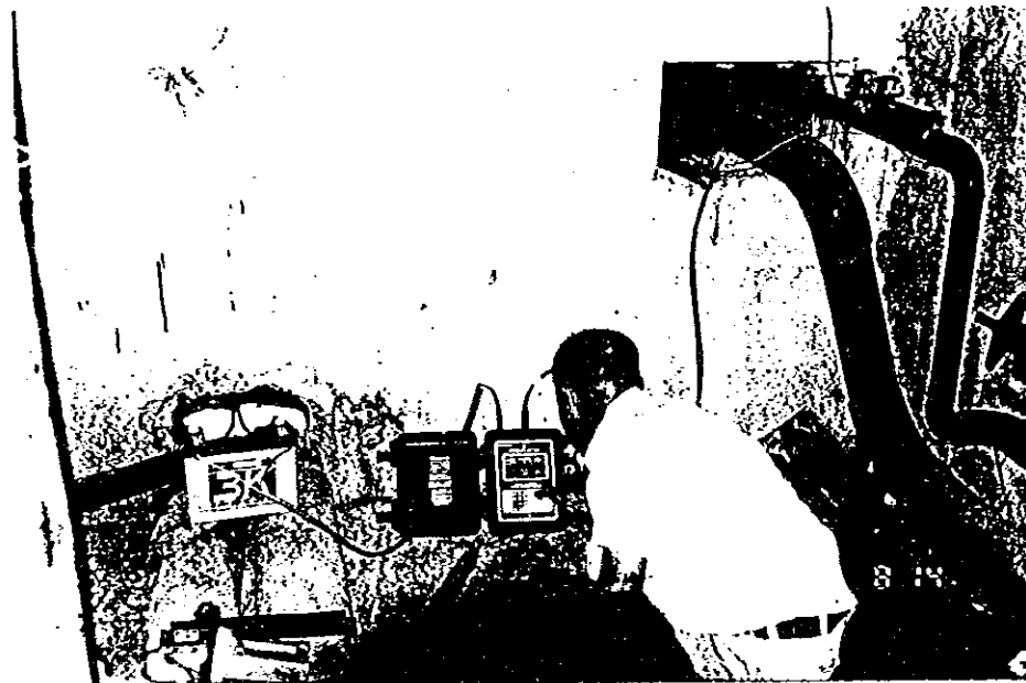
Photo 5.2.7 Ultrasonic Flow Meter in an Apartment Building
