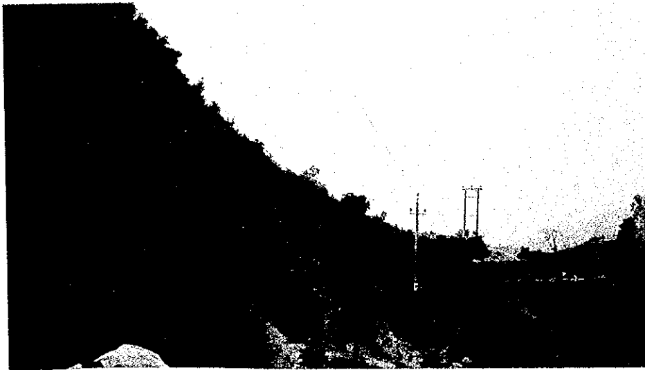
Photograph 2.3.3 Power transmission lines near Sindhuli Gadhi
