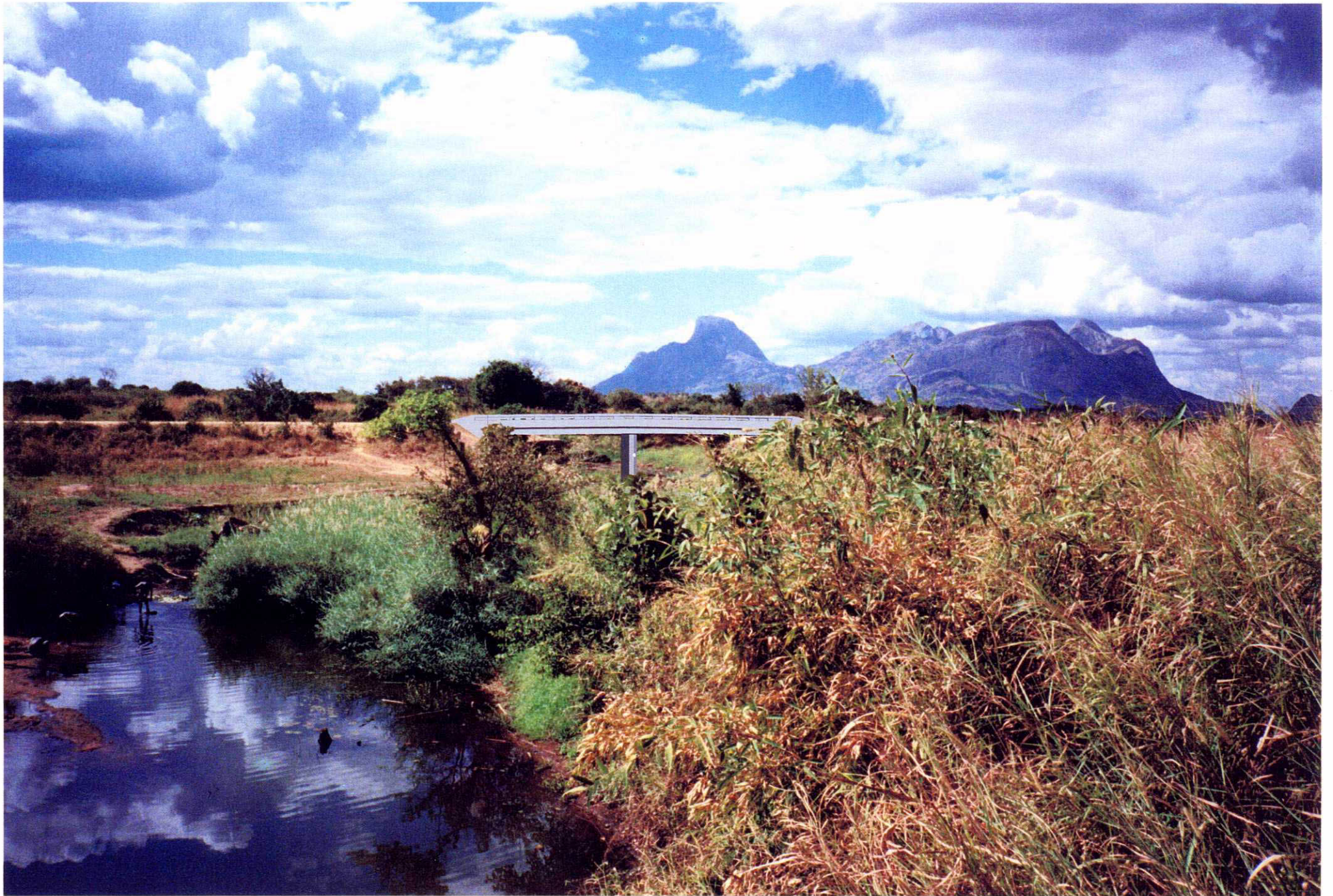
Ningare Bridge (ニンガレ橋遠望)
