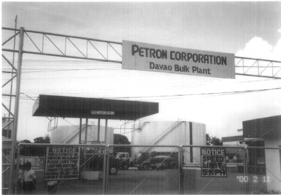
PETRON · Bulk Plant (Davao)
