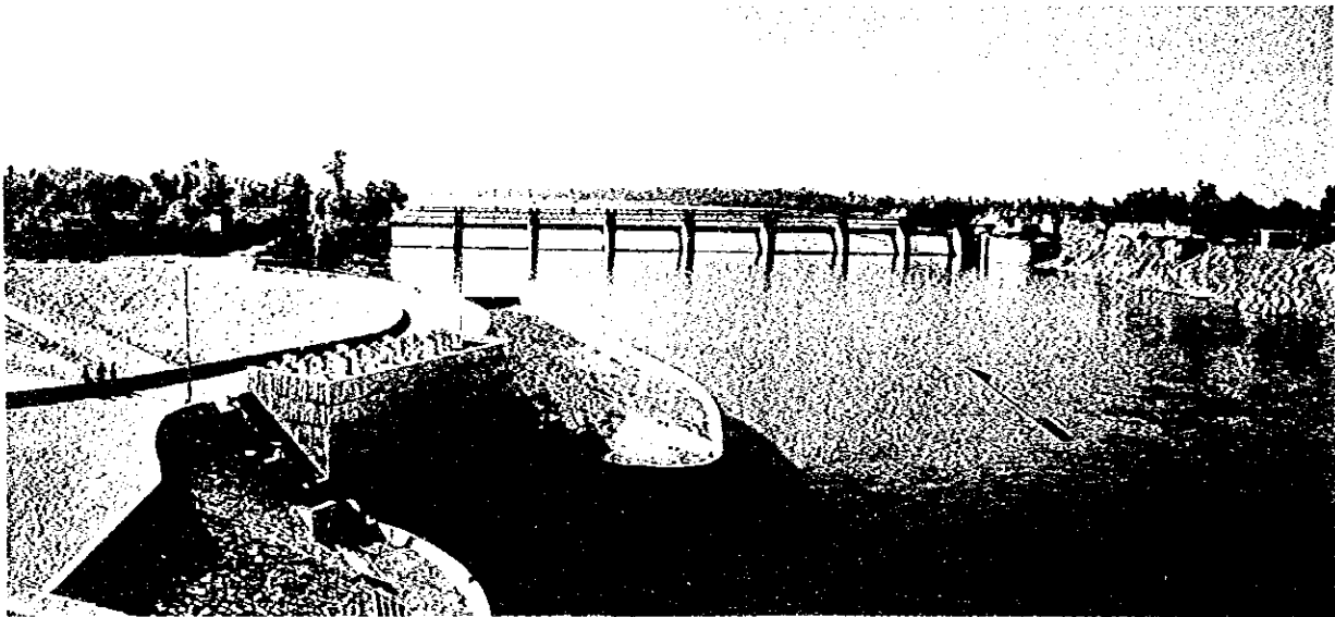
Existing Munda Headworks
