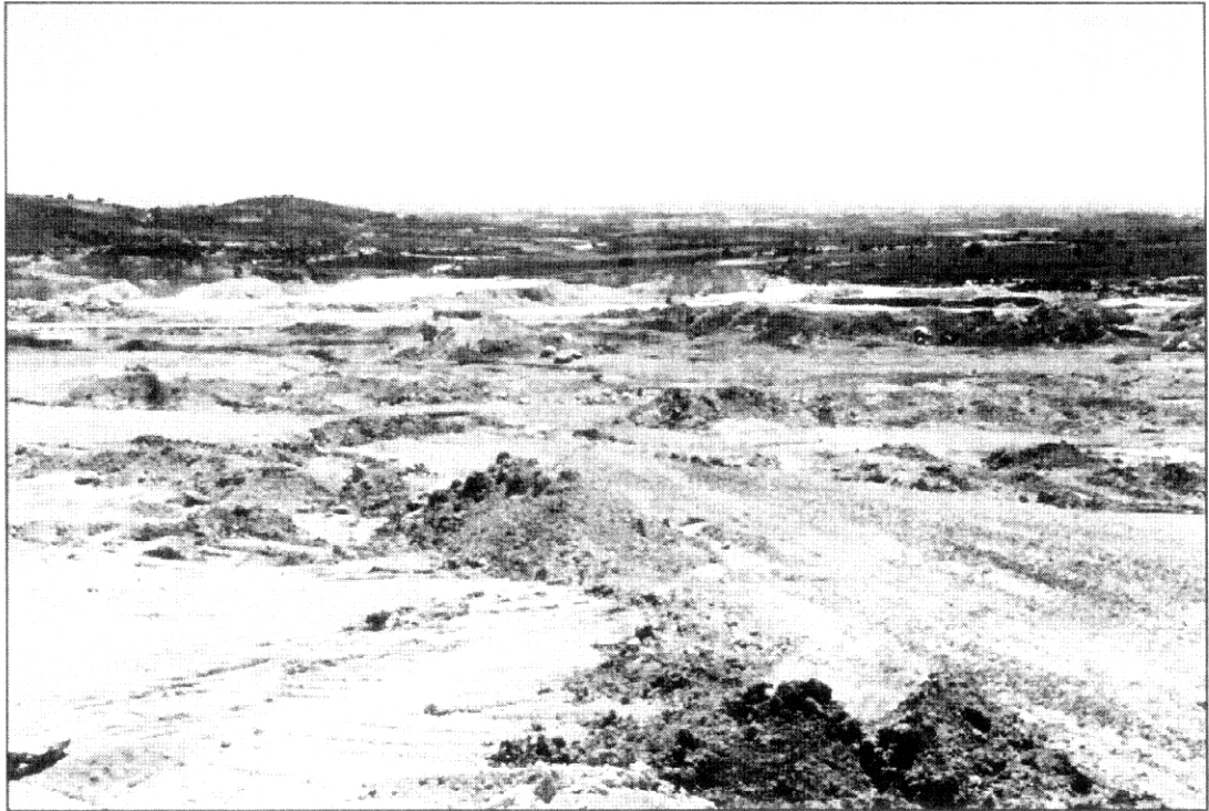
Figure 14-9: Excavation Fields in Cimsa
