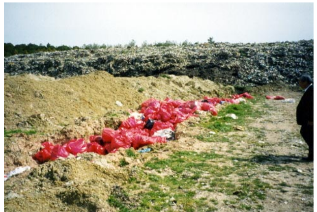
Medical wastes discharged into a trench inside Compost plant final disposal site
