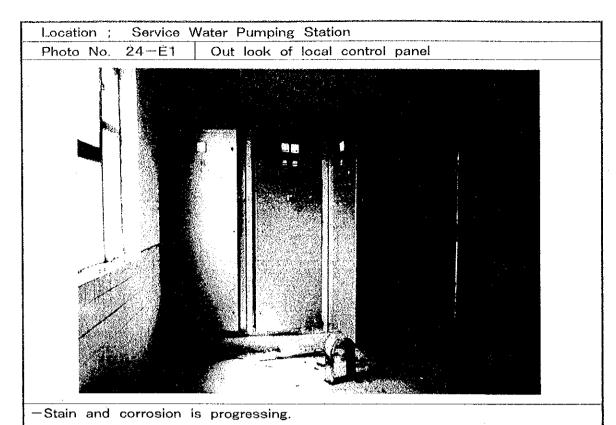
Main instruments ∕ parts were removed and taken away.All wiring and cables were cut and taken away.
