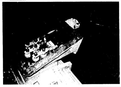
Rust is much progressing in TERMINAL BOX, and TERMINAL BOLTs are corroded.
