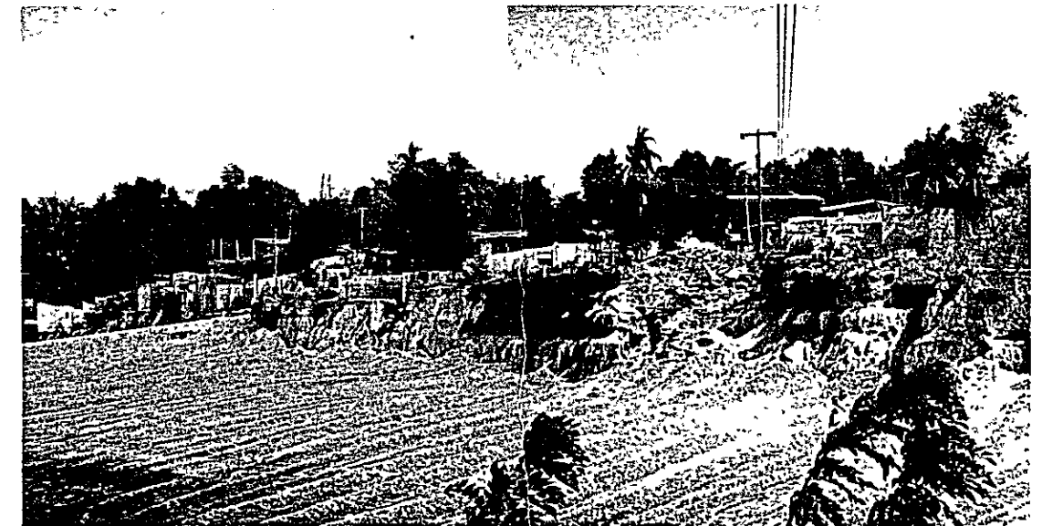
Bank erosion at Sapang Bato in upstream Abacan River (March 1993).
