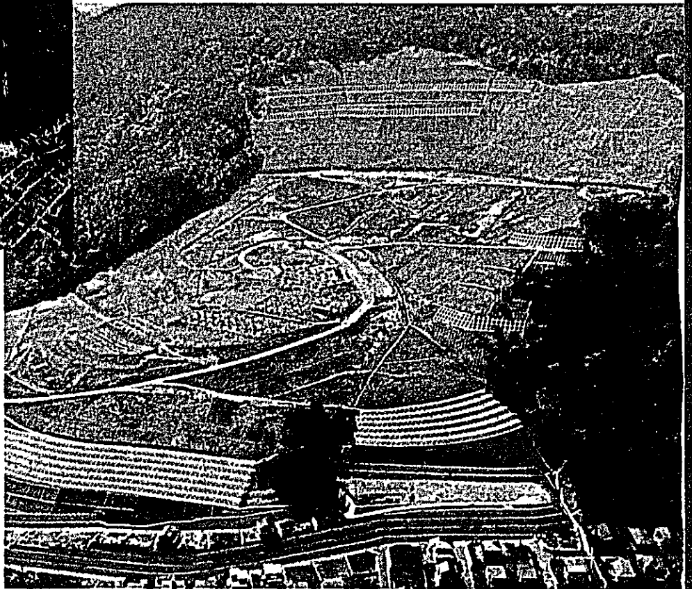
The same area after having been cleared and stabilized, with landslide control works completed for more efficient land use (Reference No. 3, page 13)
