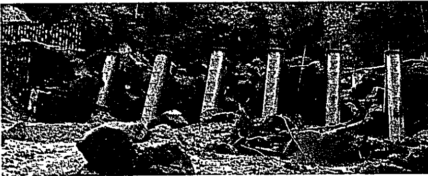
Steel Slit Dam at Mt. Usu (Reference No. 2, page 17)
