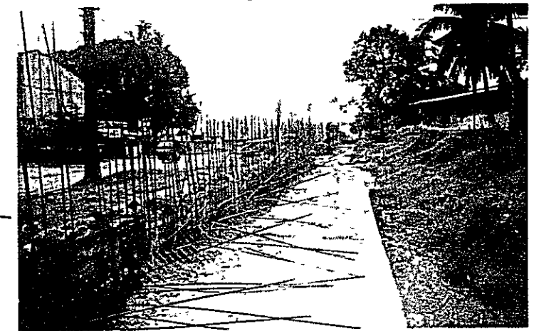
On-going Floodwall Site
