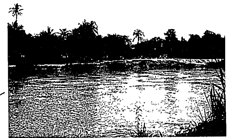
Damaged Ilog-Hilabangan River Control Project
