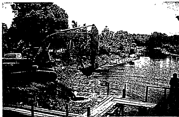
Villa Kananga Open Canal on-going deepening and widening
