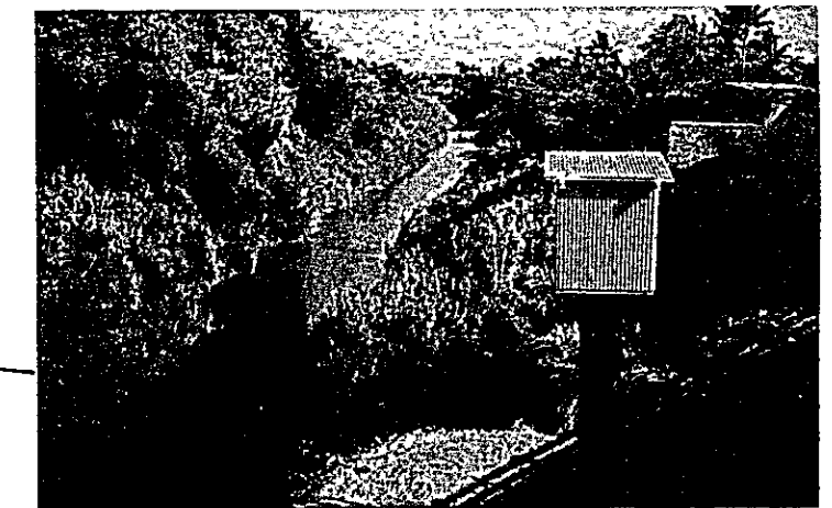
Water Level Gauge located at Jaro Bridge
