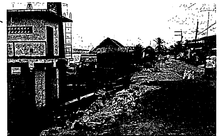
Bato Lakeshore damaged by Typhoon Rosing, 1995
