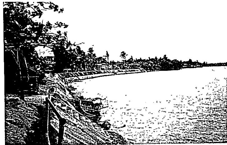
Bank Protection of Libmanan River, Camarines Sur
