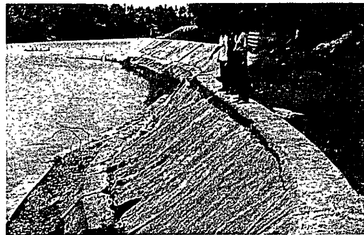
Damaged Ilog-Hilabangan River Control Project
