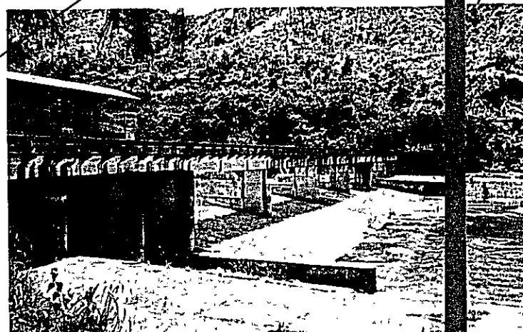
NIA Irrigation Diversion Dam in Madongan River
