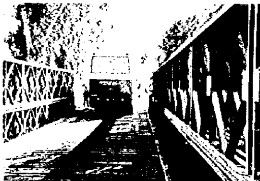
The existing Bailey bridge allows only one vehicle to pass
