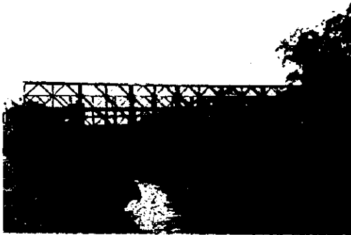
Existing King Hussein Bridge viewed from the upstream
