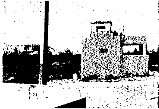
Watch tower on the Jordanian side (to be removed)
