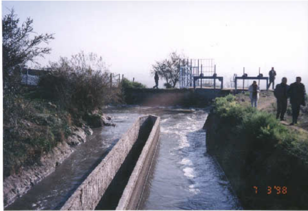
Intake facilities in the midstream of the Mapocho River (Mallarauco canal)
