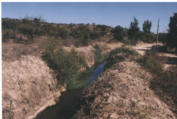
Tertiary canal without lining
