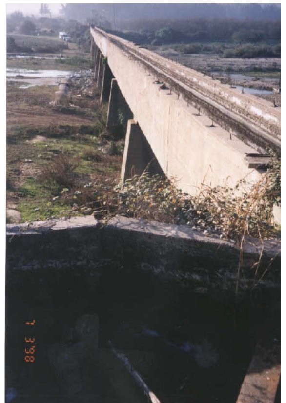
Aqueduct across the river
