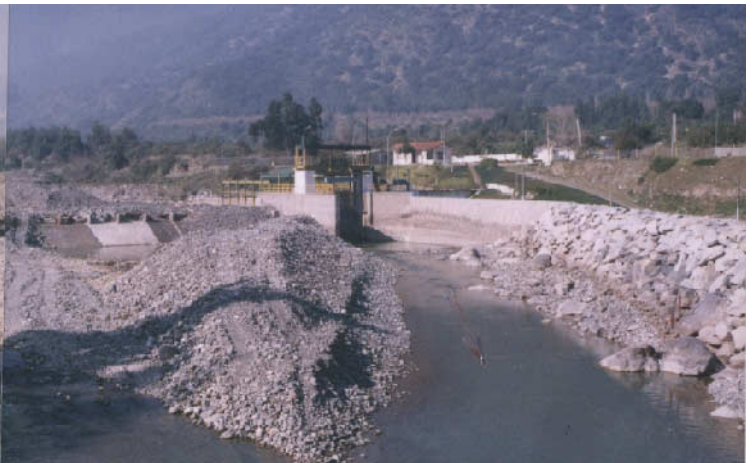
Intake facilities of the first section of the Maipo River (Obra head works) Left; San Carlos canal for agricultural use, Right; intake canal for water supply managed by EMOS
