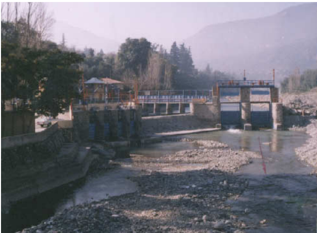
Intake facilities of the first section of the Maipo River (Obra head works) Left; San Carlos canal for agricultural use, Right; intake canal for water supply managed by EMOS
