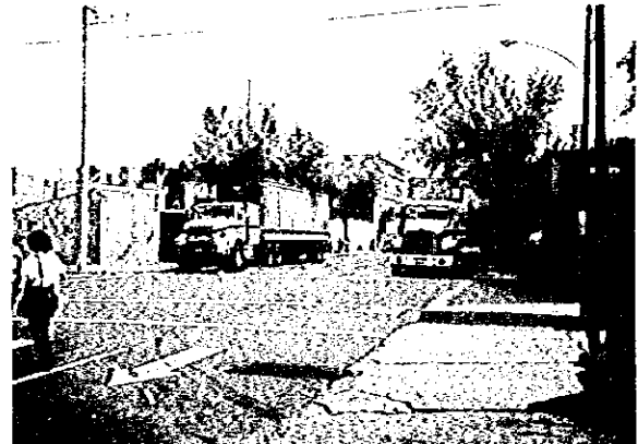
Large-size trailer (70 m 3 ) hauling waste
