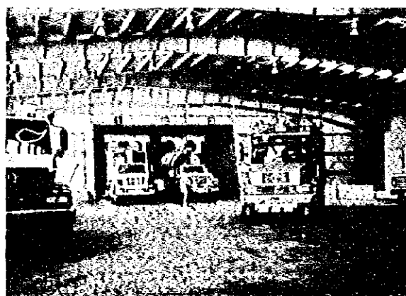
Refuse inlet of the transfer station. Waste will be transferred from collection vehicles to large-size trailers
