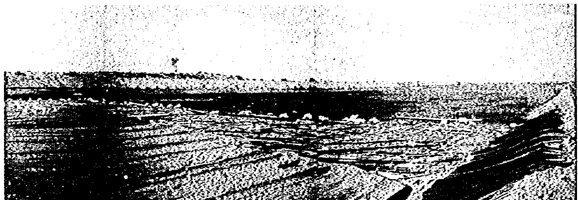
Bordo Poniente Etapa IV Landfill. The foreground shows a future cell being under construction of impermeable liner. The distant view presents a cell being currently filled.
