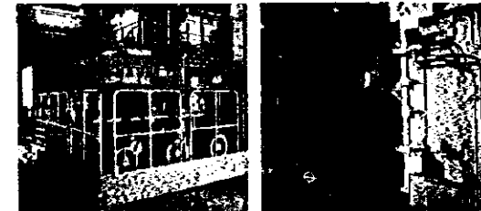
⑥ Hydraulic power unit ⑦ Cleaning device to wash off refuse stuck to container tailgate
