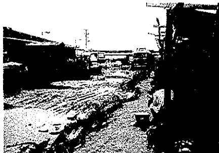
② ■ The muddy condition of the unpaved road after a rain.
