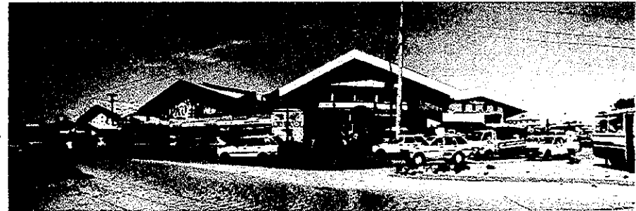
① ■ The building on the right was extended by the Cooperativa.
