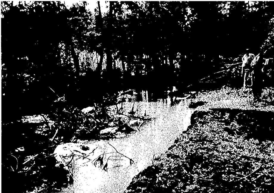
Simple intake facilities provided by tree and embanked soil in Ngomano/Nyangati Water Furrow Project. Intake is washed away every year by flood.
