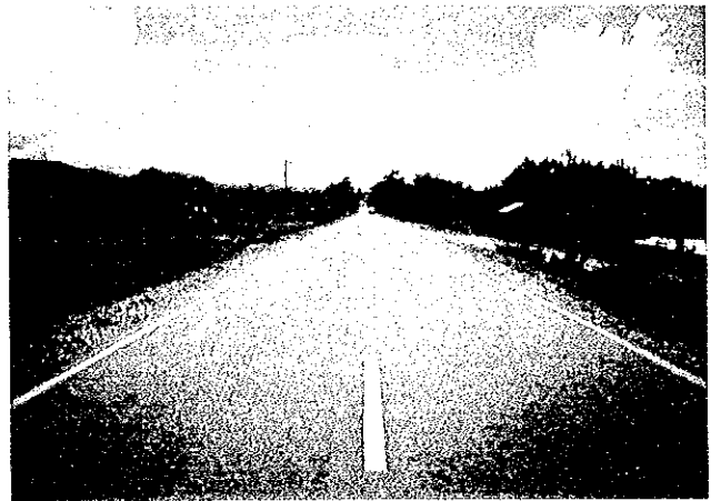
AC Pavement in good condition Sindagan - Leon Postigo( Bacungan ) Road, Zamboanga del Sur
