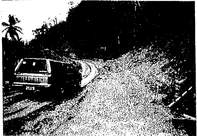
Earth road in bad condition Leon - Bucari Road, Iloilo
