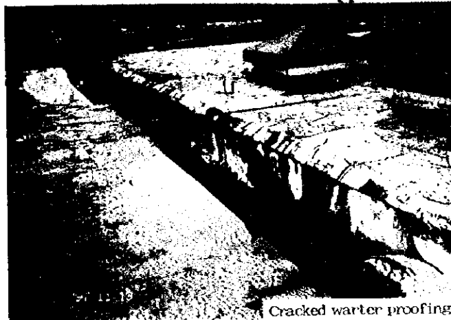
Cracked water proofing
