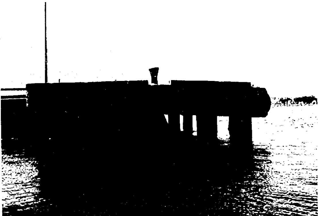
Photo - 10 Existing Wharf (North End)
