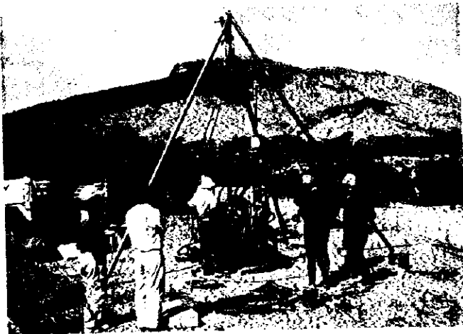
Boring Test at the Pumping Station (Block D)
