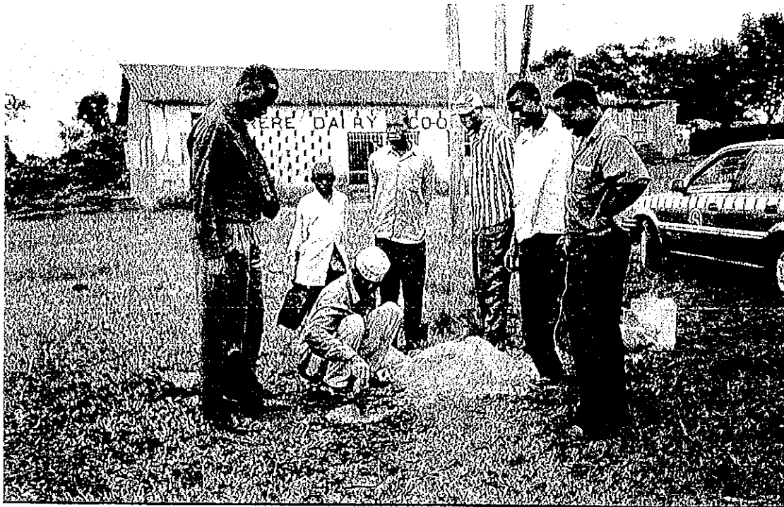
Plate 4 Backfilling the holes
