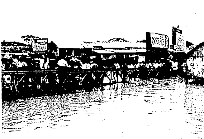
Photo-3 : Access Bridge at Rupsa Ferry
