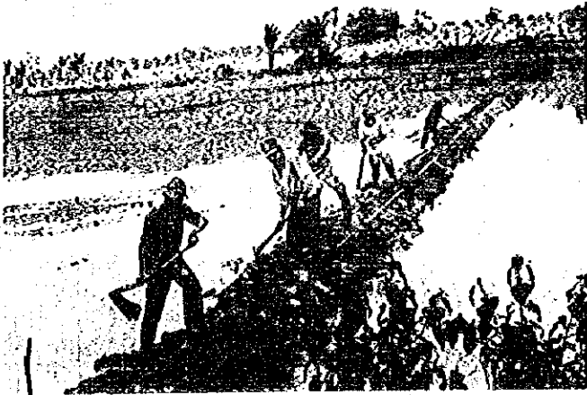
Paddy field construction work in Lalobao; Terminal irrigation ditch was constructed by farmers group work
