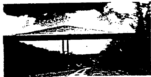
Barton Creek Bridge
