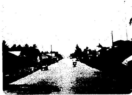
National Highway No.1 (Can Tho to Ca Mau)
