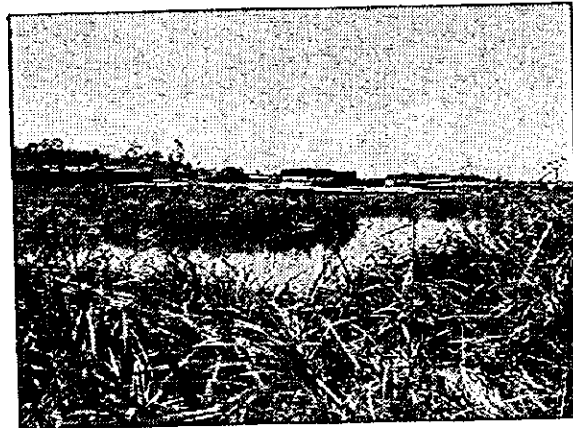
Primary Waste Stabilization Pond: note heavy overgrowth
