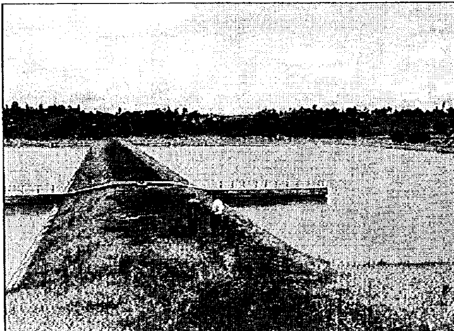
Facultative Ponds: note inter-pond connections, influent runs underground down the middle of the embankment.
