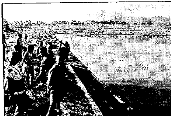
Secondary Facultative Pond: note children playing near overflow weir
