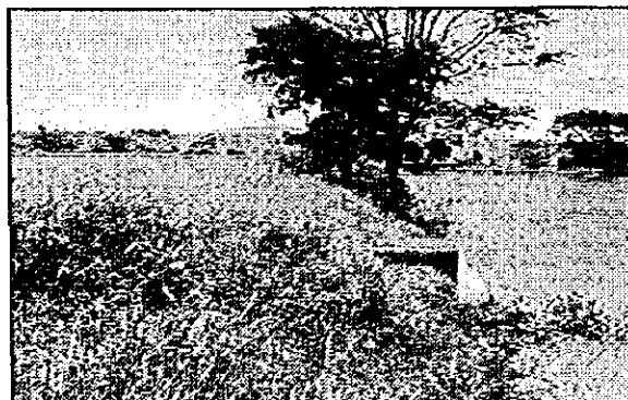
Secondary Facultative Pond: note hydraulic surcharge conditions at interconnection chamber, tall grass and trees, poor embankment maintenance.
