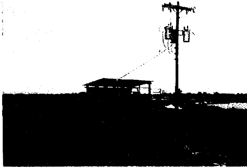
Region IV (Granada Department): Pumping station at the Malacatoya near the Lake Nicaragua, mainly used for paddy fields. The stations are generally owned by big-scale farmers and installed with a proportion of one station for about 100 hectares.
