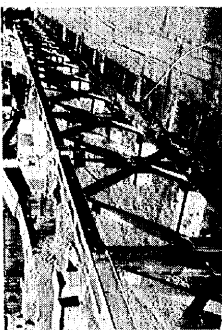
Rusty members. This pier was replaced, when buckling occurred.
