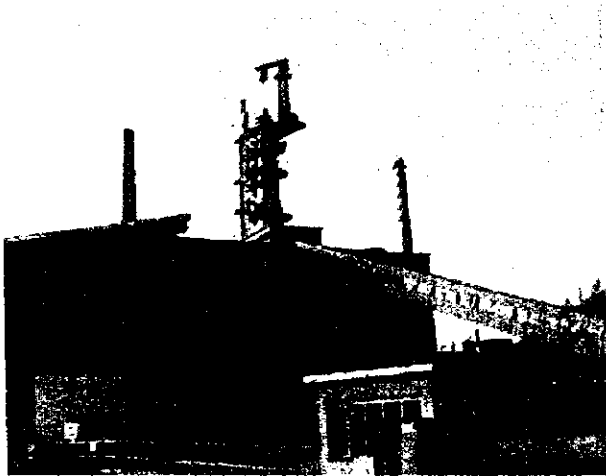
9) Chip conveyor, storage and kamyr digester
