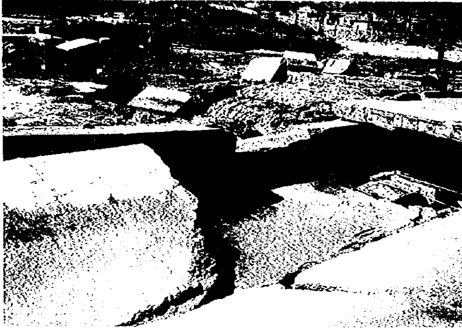
Photograph (7) Damaged Anchor Concrete Block ( Wharf)
