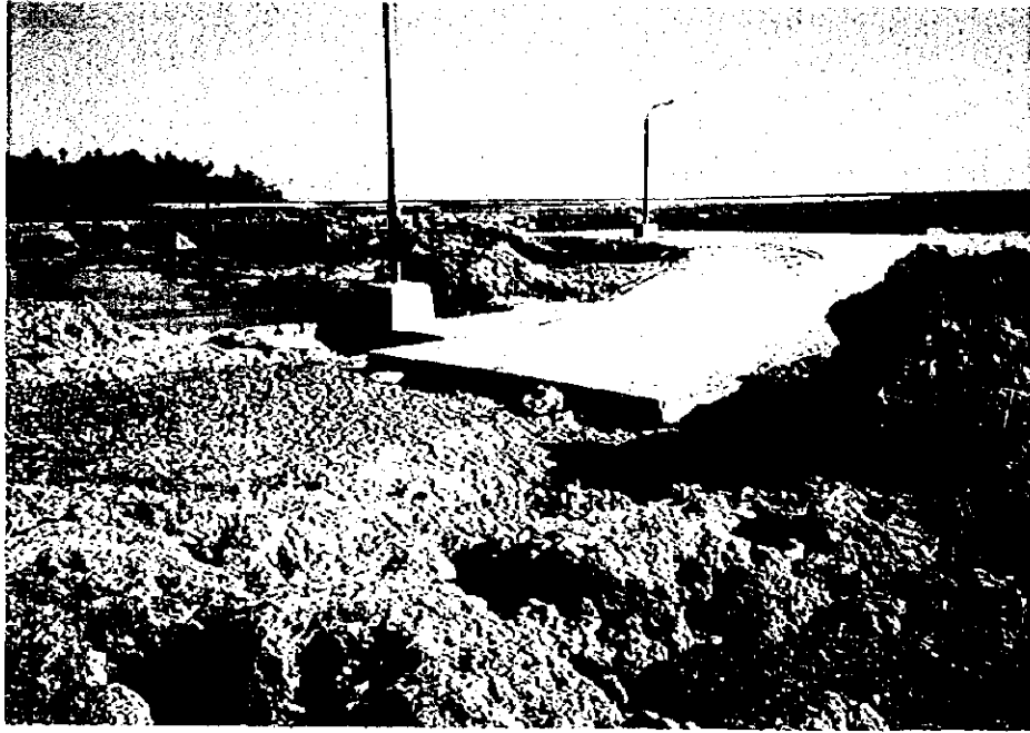
Photograph (3) Damaged Access Road (Transition from concrete to gravel pavement)
