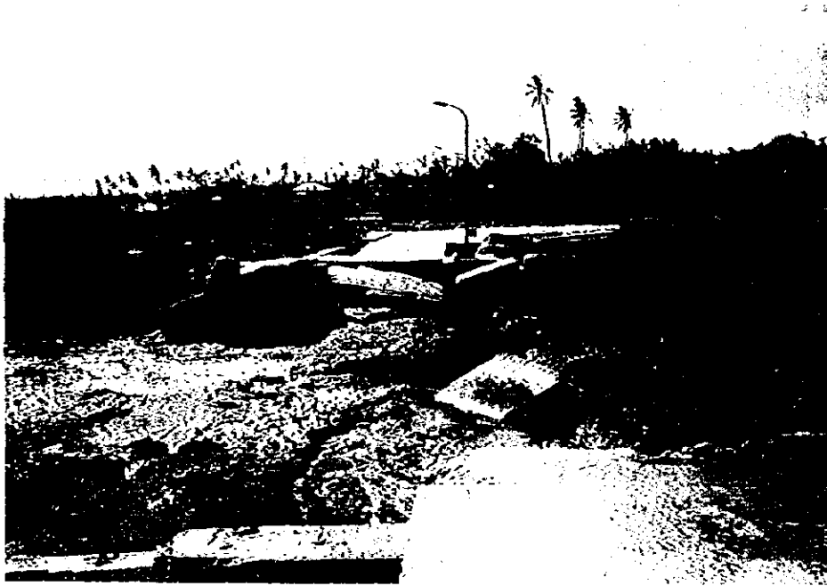
Photograph (5) Access Road Washed Away ( Area of Connected to the Wharf )
