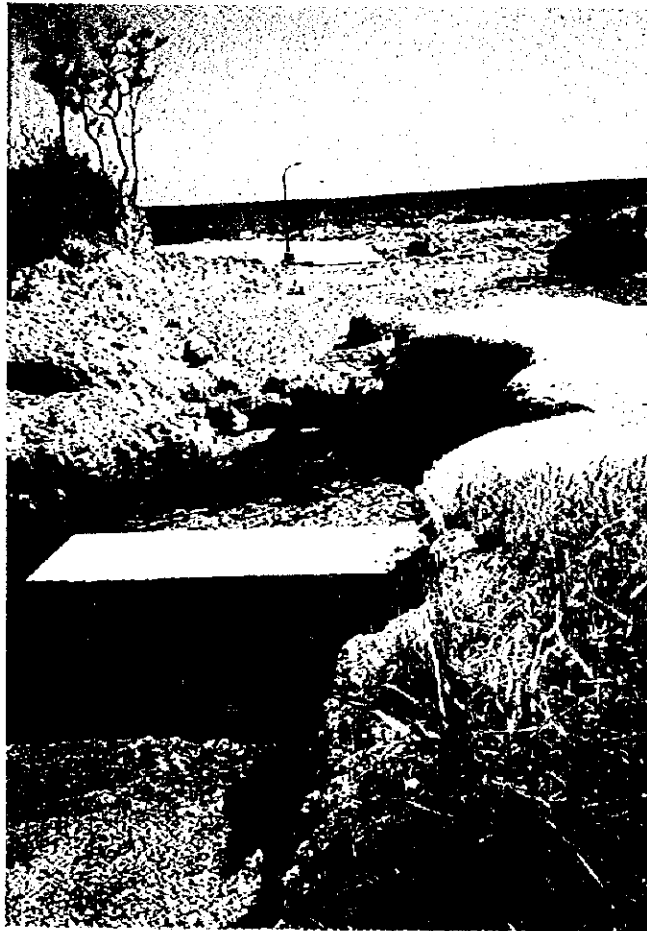
Photograph (2) Damaged Access Road (Gravel Pavement Area)
