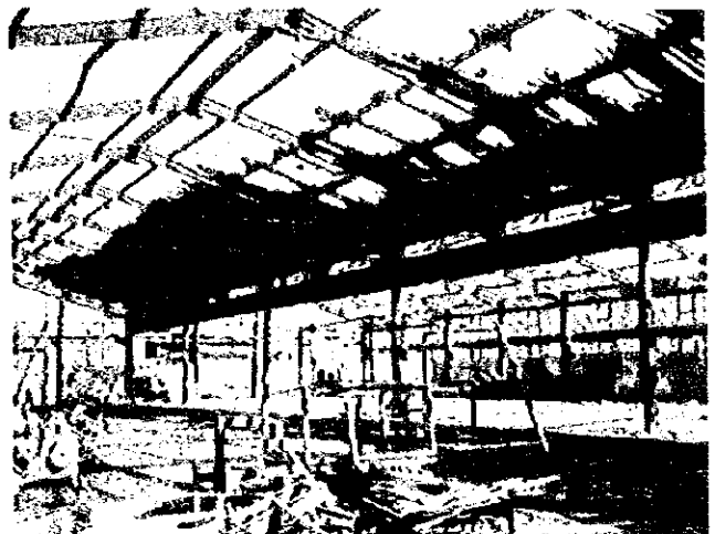
30) Burn-out corrugating section
