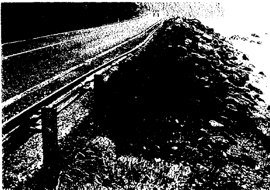
Erosion by wave action
