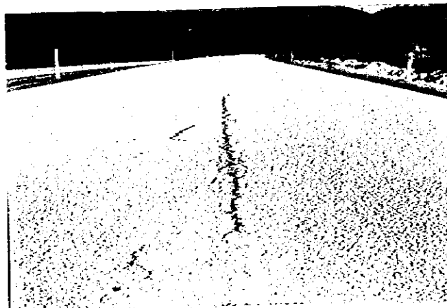
Longitudinal Cracking, Damage Rank B
