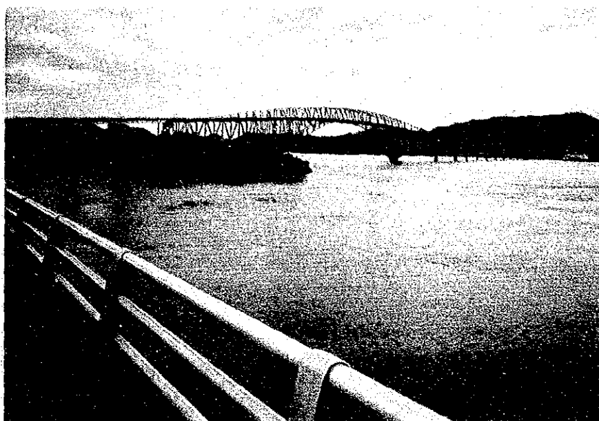
Fan Fanico Bridge (Between Samar Is. to Leyte Is.)
