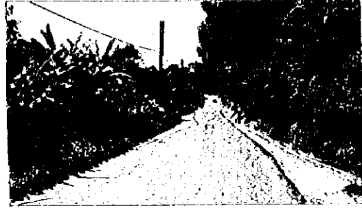
Unfinished shoulder on rehabilitated section
