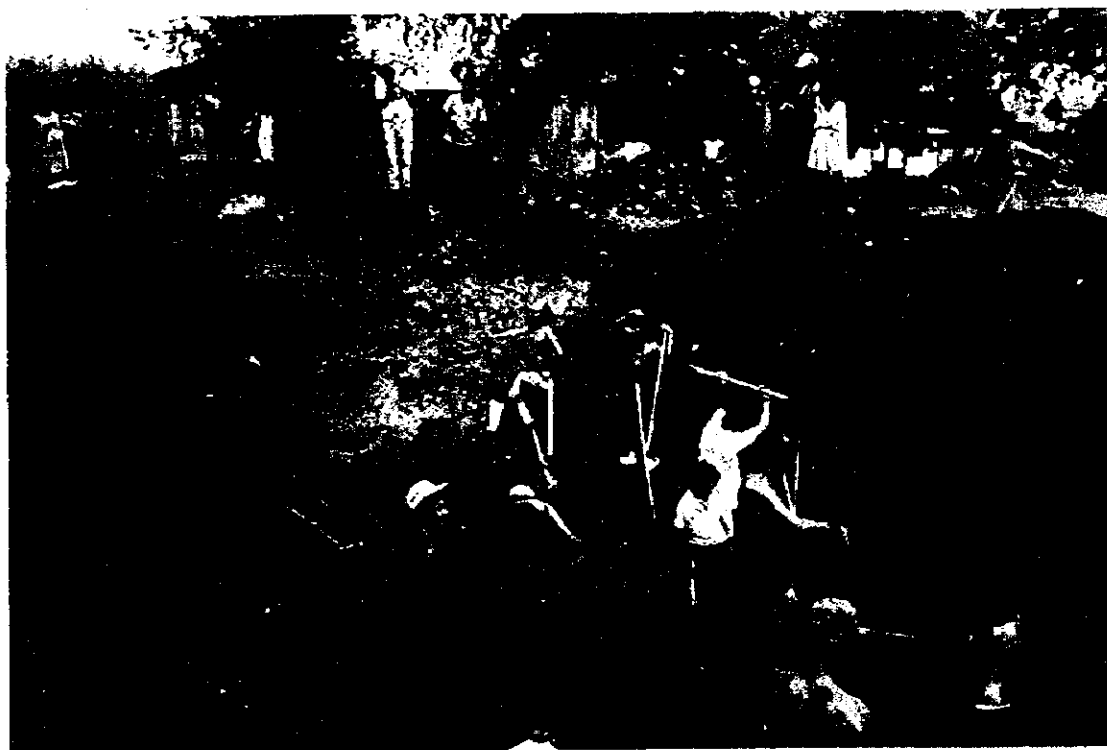
Plate O-67 : Excavation (Septic Tank)
