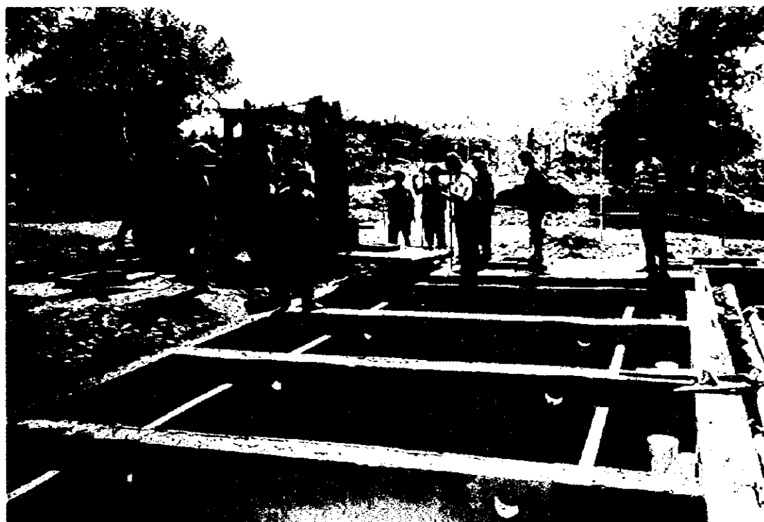
Plate O-75 : Installation of Septic Tank Cover
