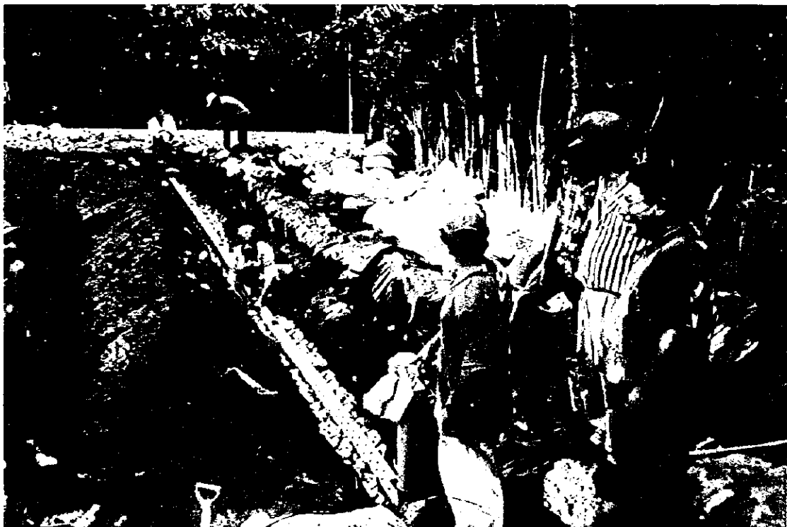
Plate O-79 : Installation of Distribution Pipe
