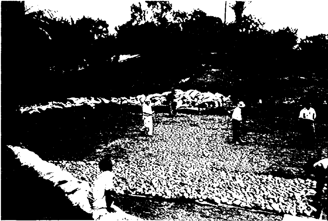
Plate O-78 : Spreading Cobble Stones (Filter Trench)
