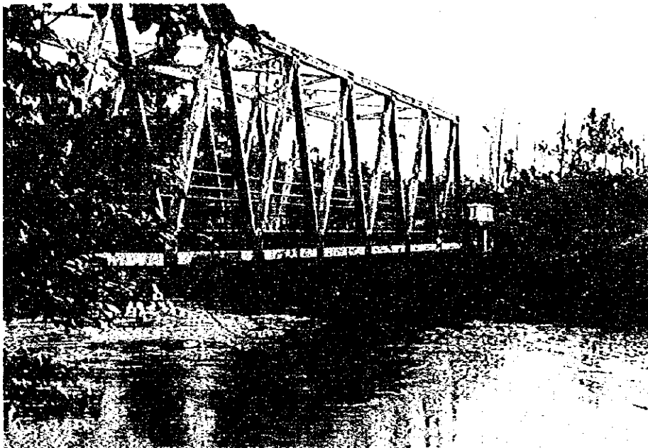
Samal River Samal Road Bridge (Flood Flow)
